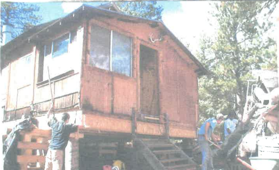
PHASE TWO - CABIN RAISED 4 FEET TO PROVIDE NEW FOUNDATION - OCTOBER 2008
