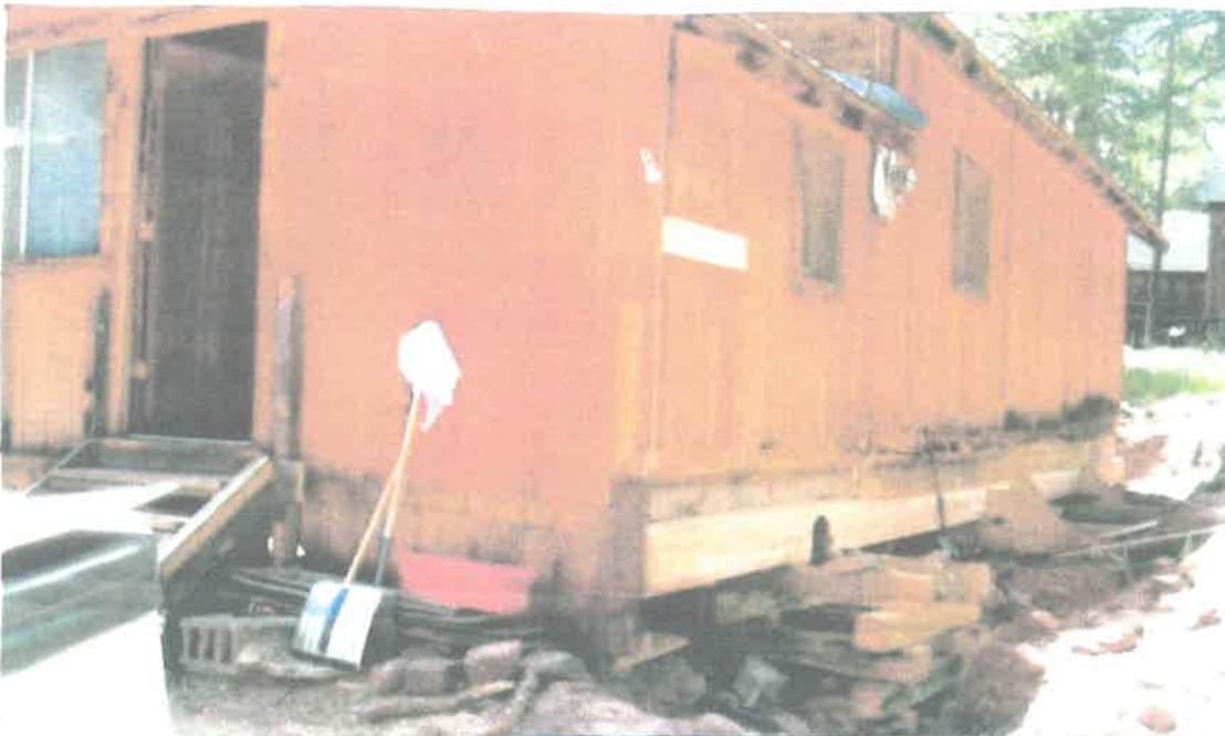
PHASE ONE OF REMODELING AUGUST 2008
